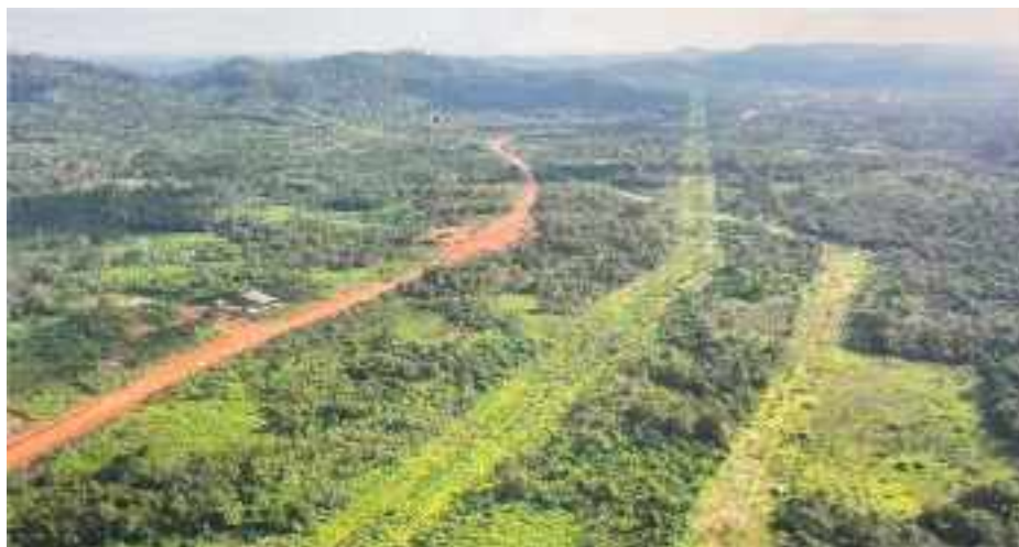
Figure 2: Access to the proposed Dunkwa II Substation
